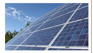
A 60-module, 16.8 kW grid-connected photovoltaic system provides the homes energy for hot water, electricity and space heat. The system is remotely mounted and incorporates a tracking system to substantially increase electricity production. Annually,
